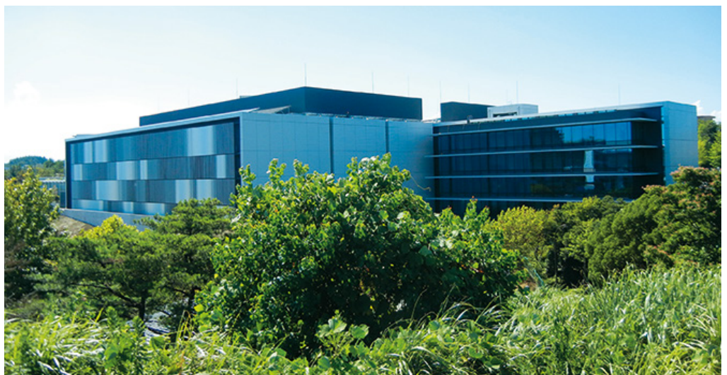
NRI's Data Centers are environmentally progressive
