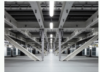
The double-decking layout, which is about 4 meters high
